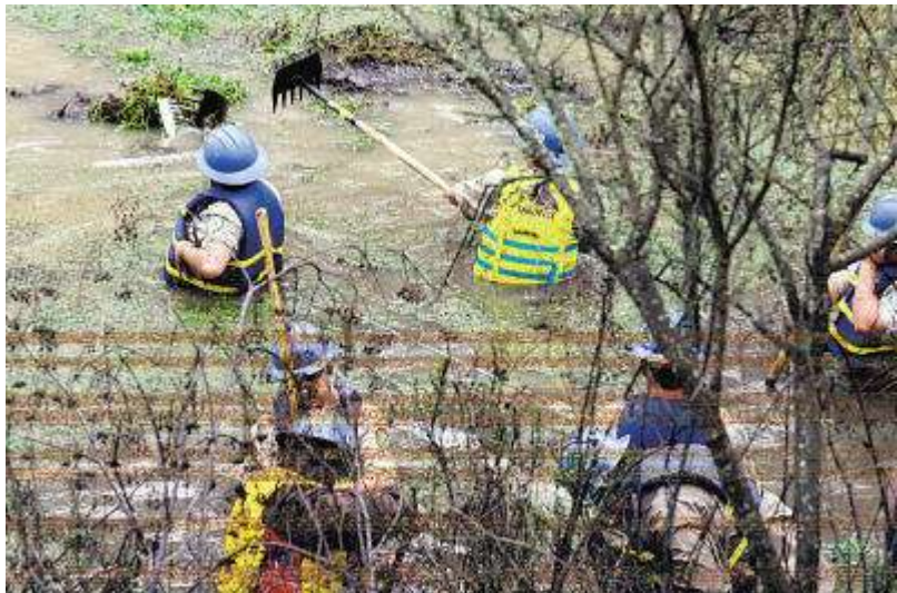
California Conservation Corps members find themselves up to their waists in Pinto Lake on Monday as they clear vegetation to open a channel (Shmuel Thaler/Sentinel)
